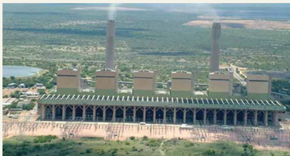
Figure 4: Matimba 3990 MW direct dry-cooling coal power plant. Eskom, South Africa (Eskom 2013).
