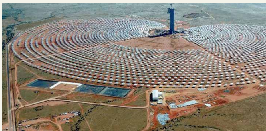
Figure 12: Khi Solar One: 50MW central receiver. Abengoa, South Africa (Abengoa 2014b).
